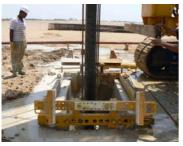
Construction of the barrettes using hydrofraise and bentonite slurry
