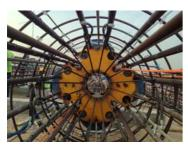
O-cell Assembly in Working Pile
